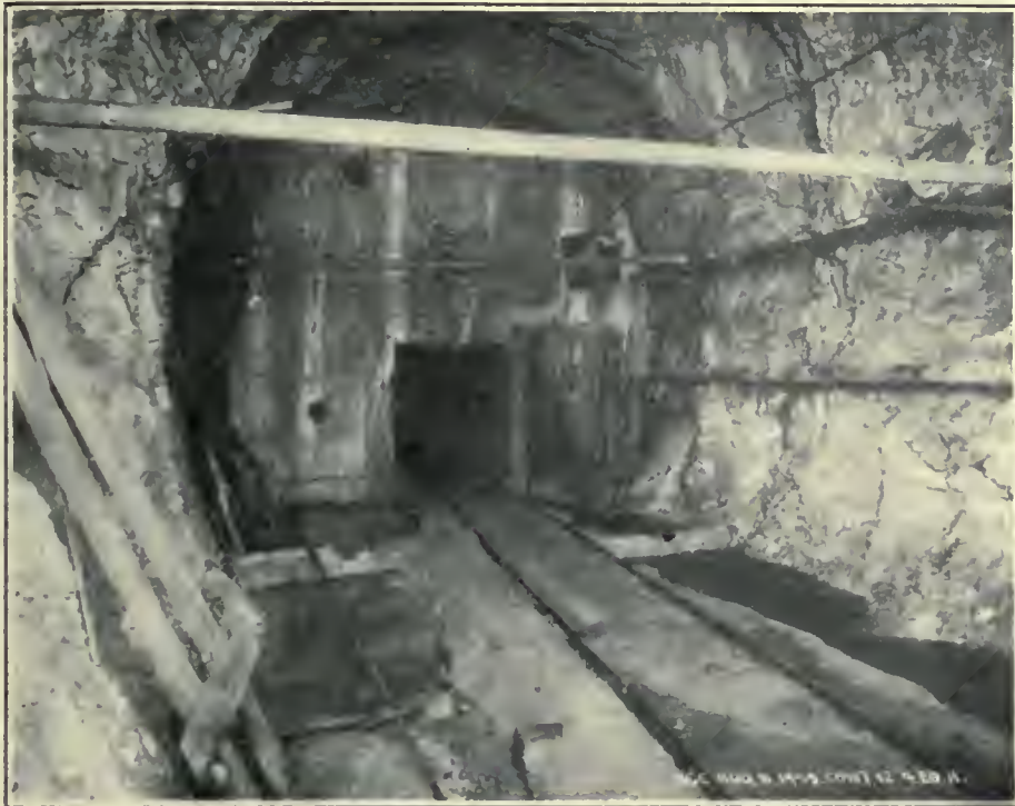
CONCRETE BULKHEAD NORTH OF SHAFT NO. 4.
